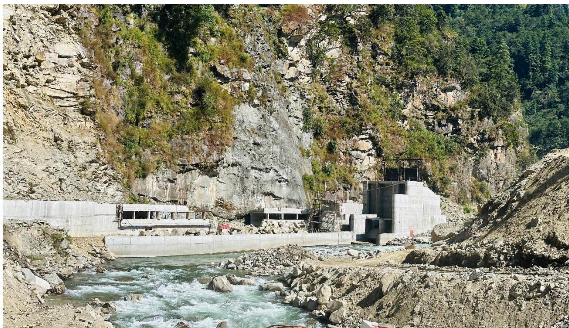
Flood wall, approach culvert & intake
