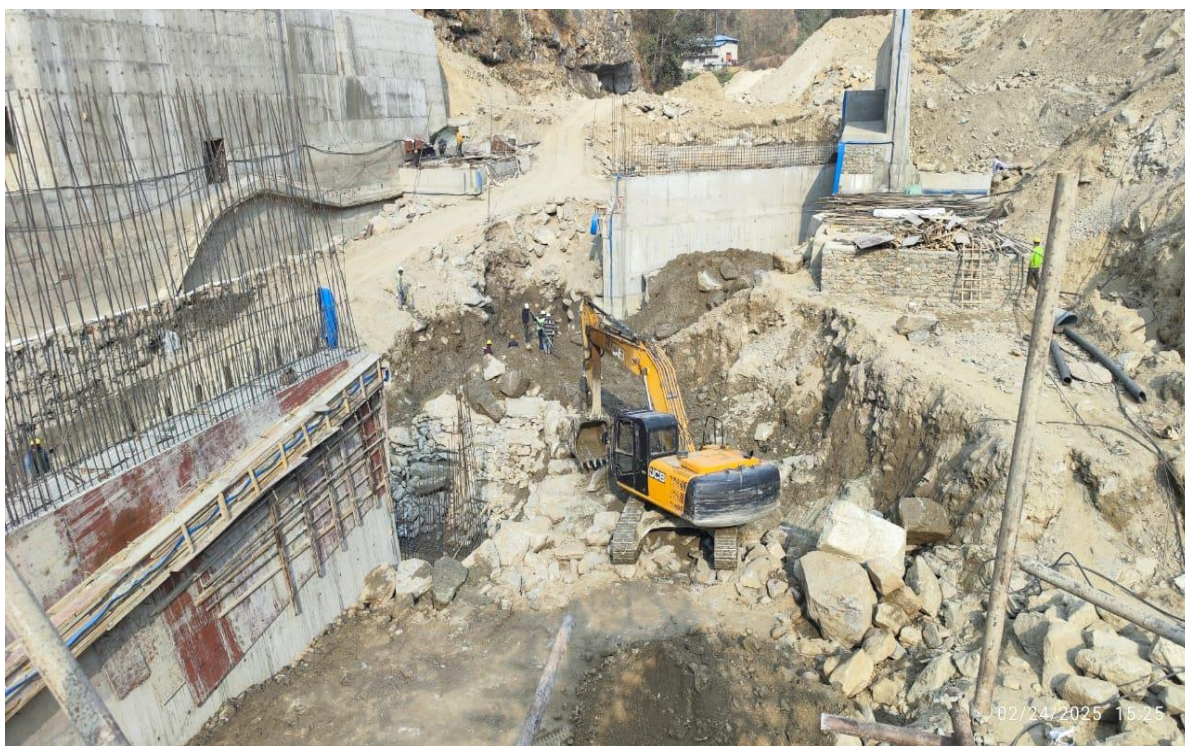
Base preparation on ogee shape spillway
