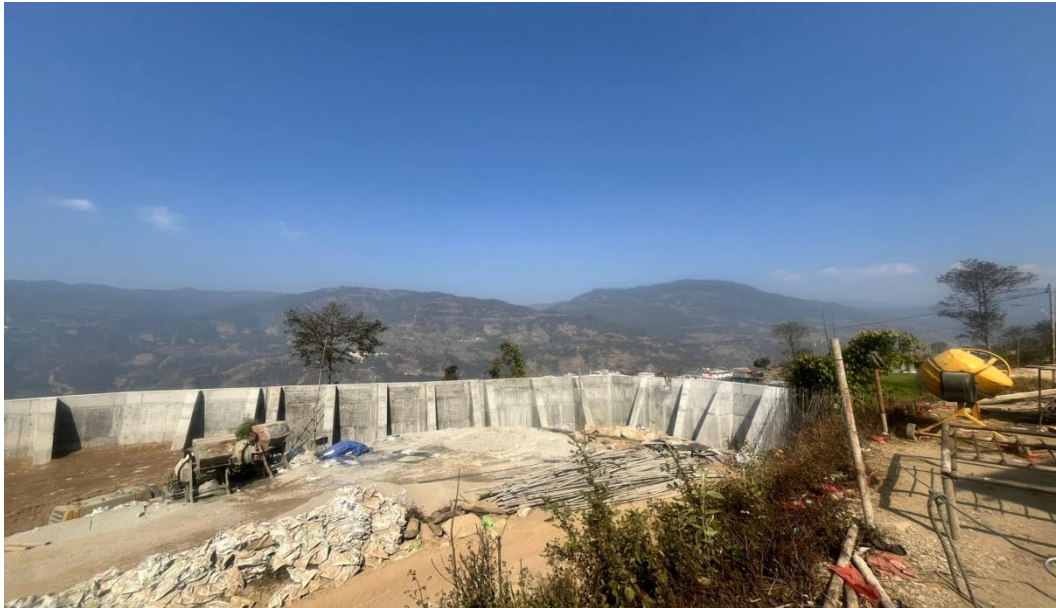
Masonry work, R.C.C work and Back fill
