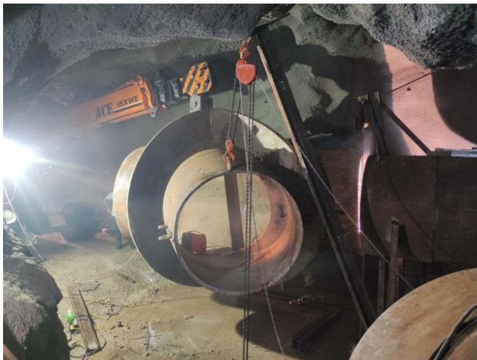
Bifurcation-I Erection Works
