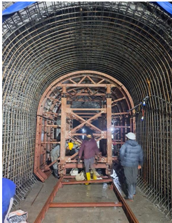
Lining works from Face 2 (Invert, wall and arcs)
