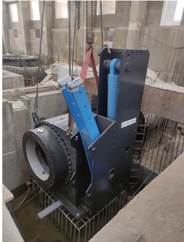
Installation of Unit 3 MIV
