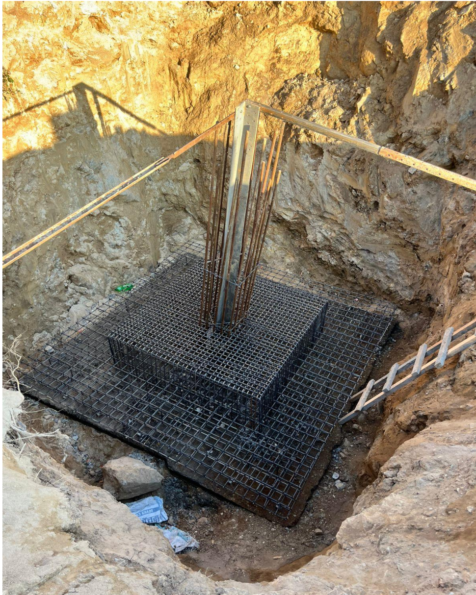
AP 7 foundation works
