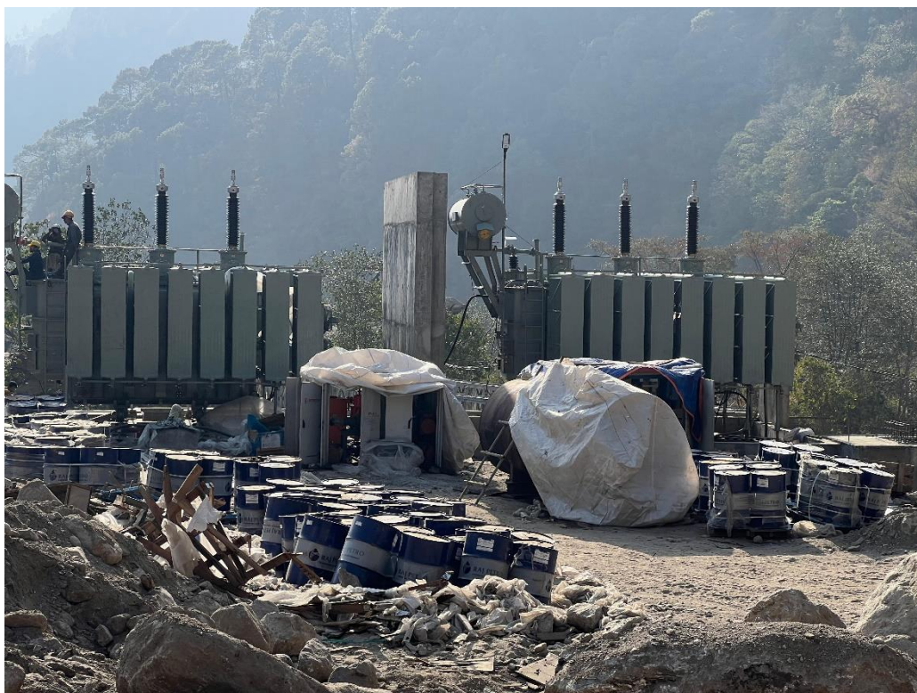
Installation of Power Transformers
