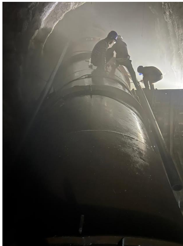
Drainage Pipe Installation at UPT
