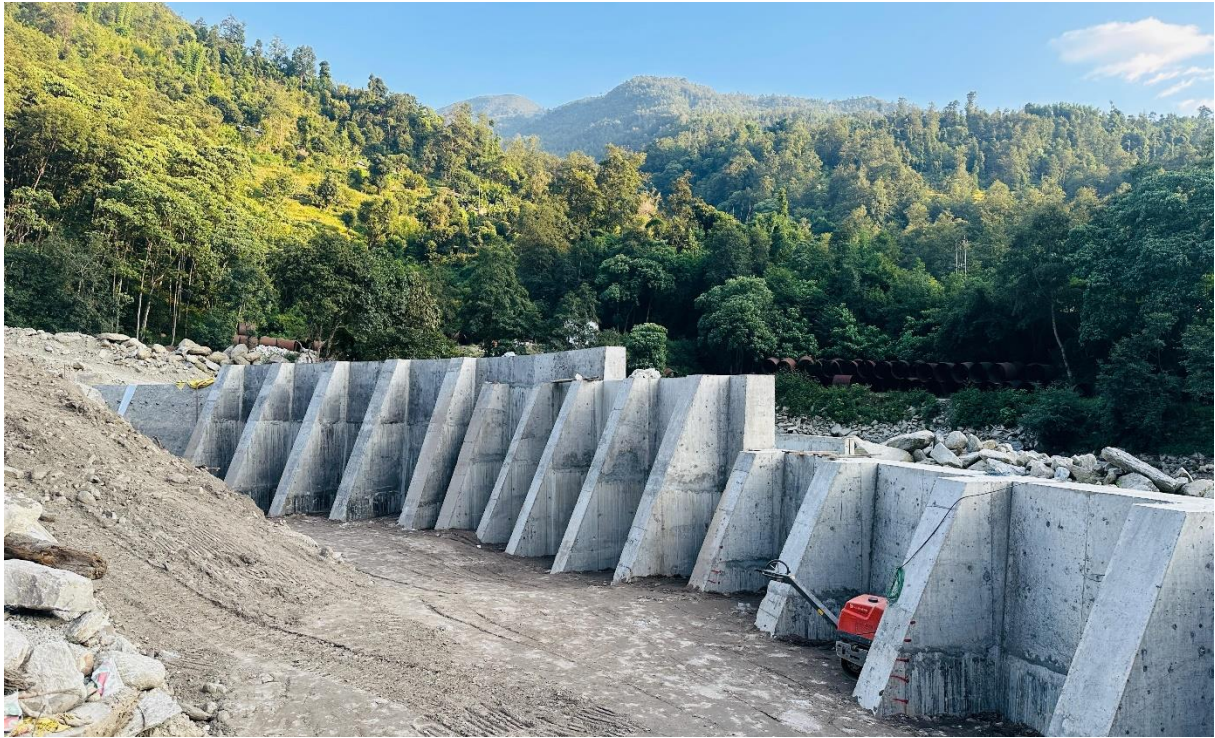
Switchyard Retaining Wall
