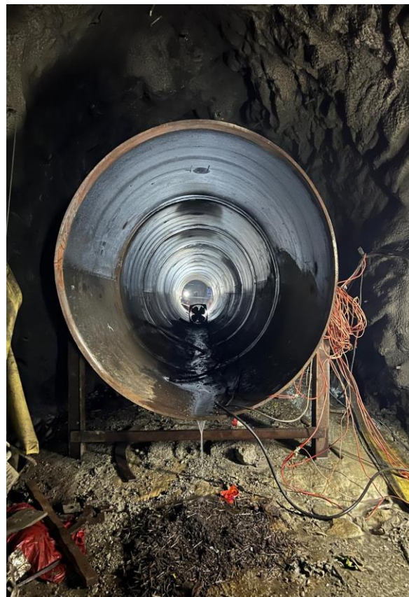
UPT Pipe Erection
