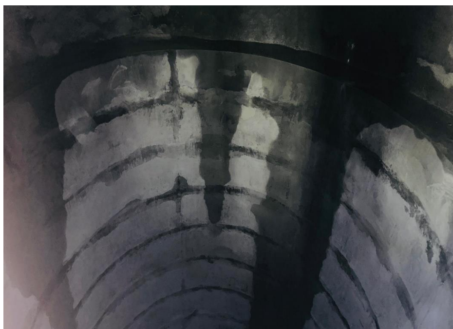
Surge shaft concrete works completed
