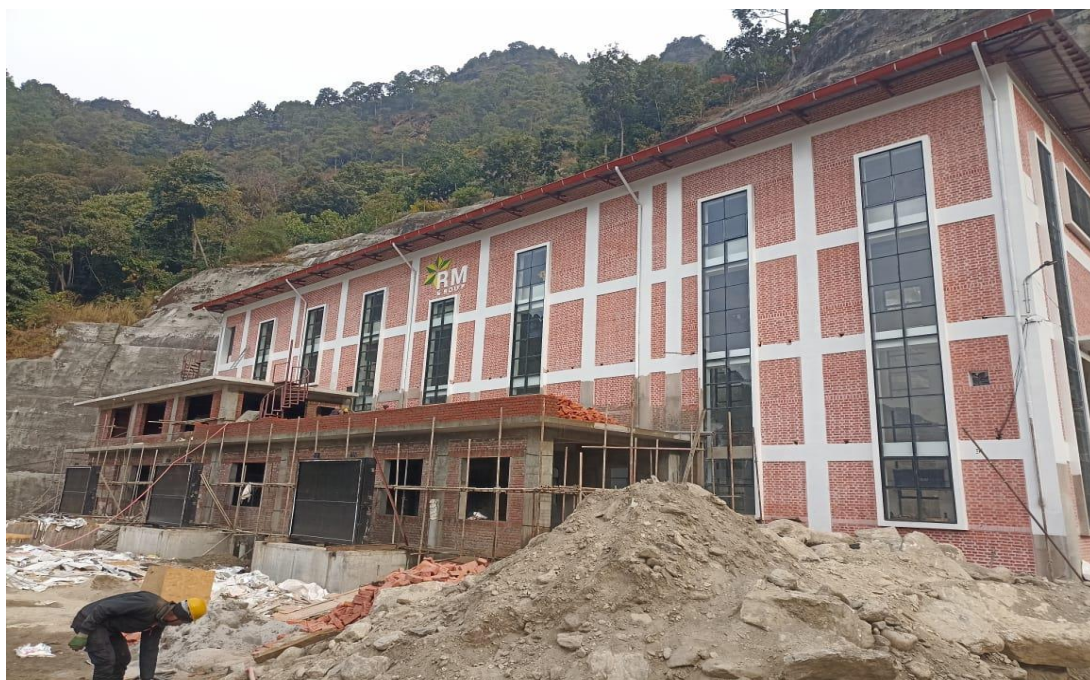
Powerhouse & Control building
