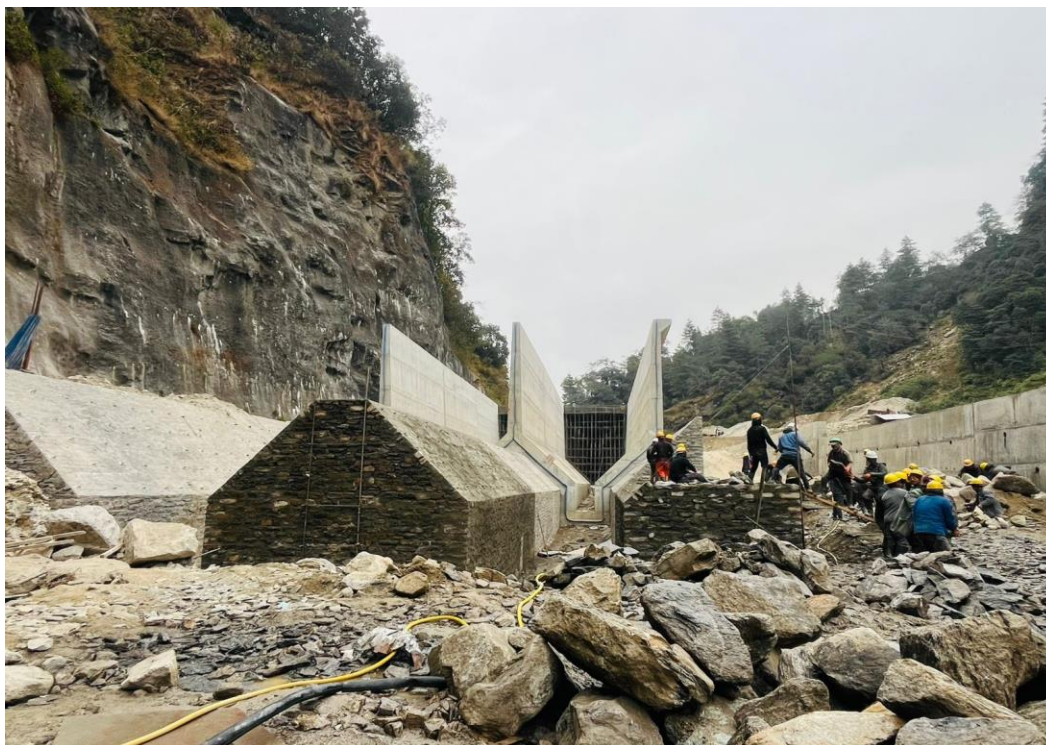
Settling basin (masonry wall)
