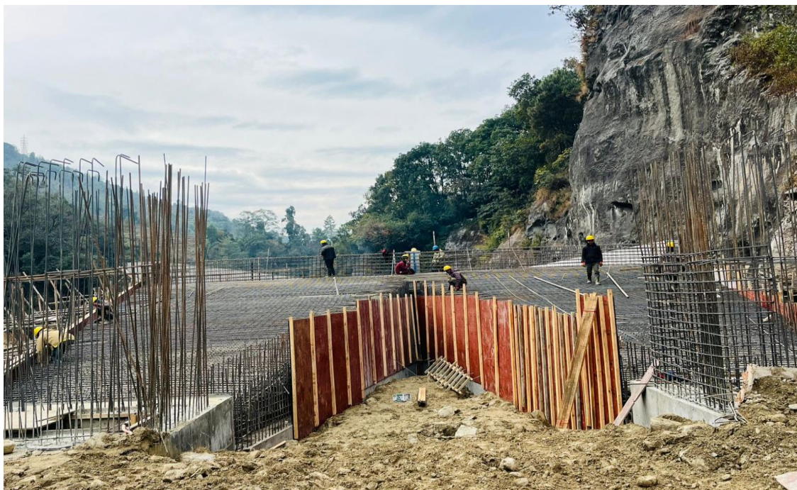
Rebar & form work at transition part(slab)
