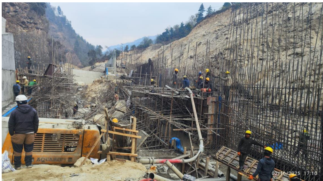
Rebar & form work at transition part(slab)
