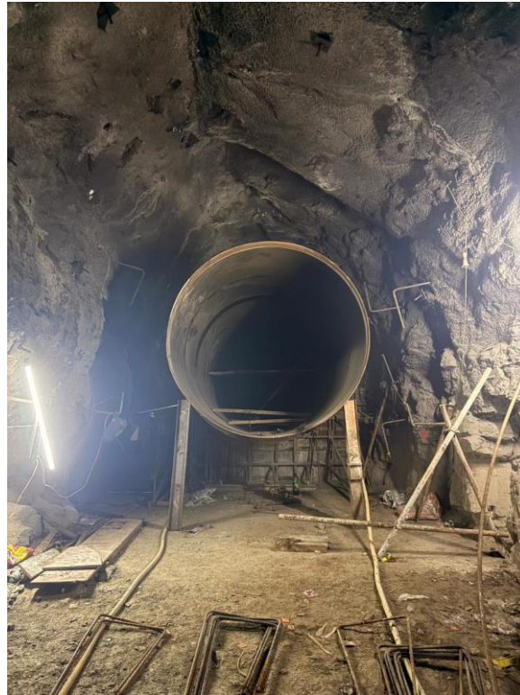
Pipe Erection at Surge
